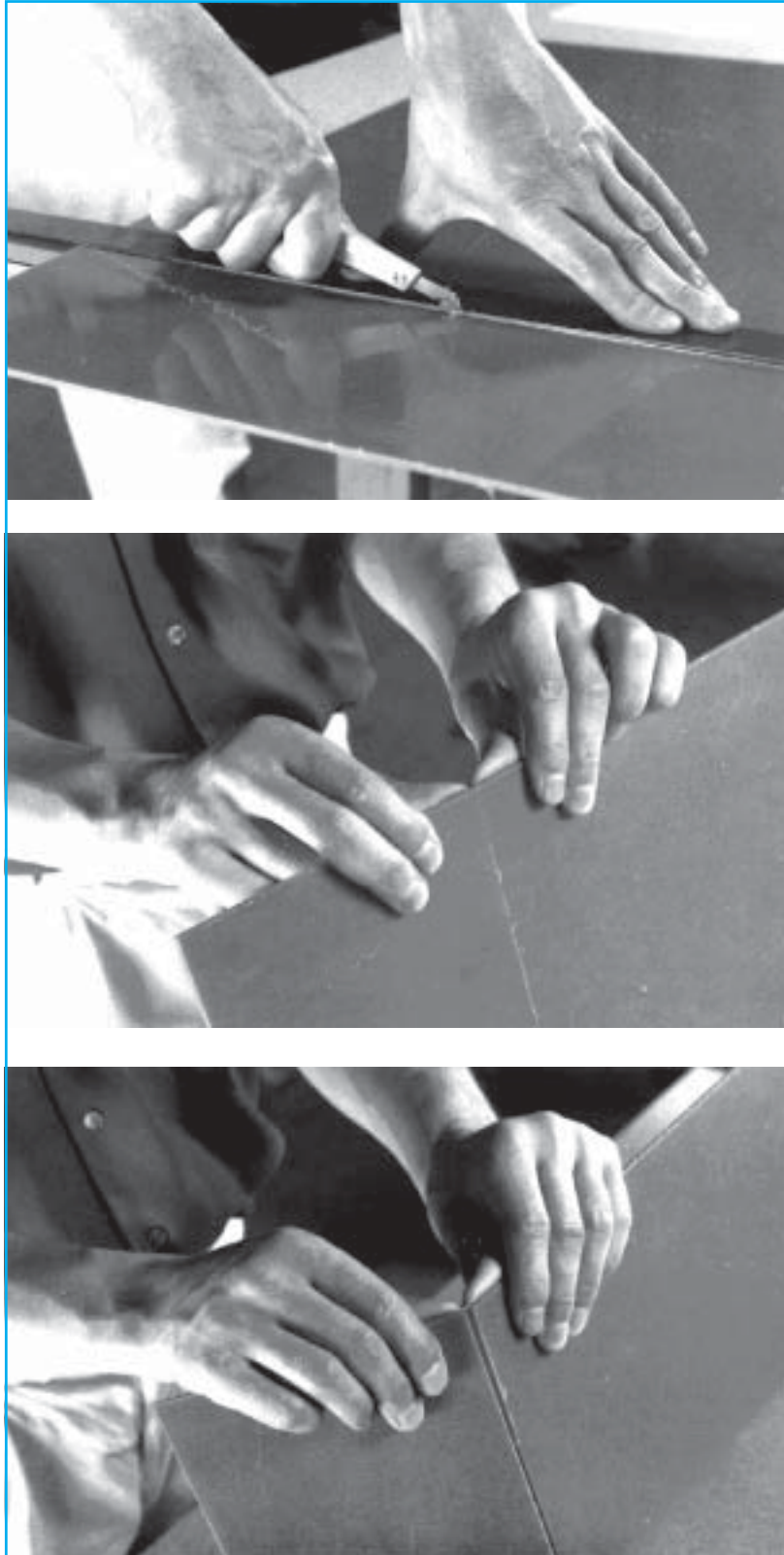
Fig. 11: Scoring and breaking
